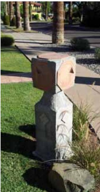
A stucco finished the column, and a final grout can be used if so desired.
