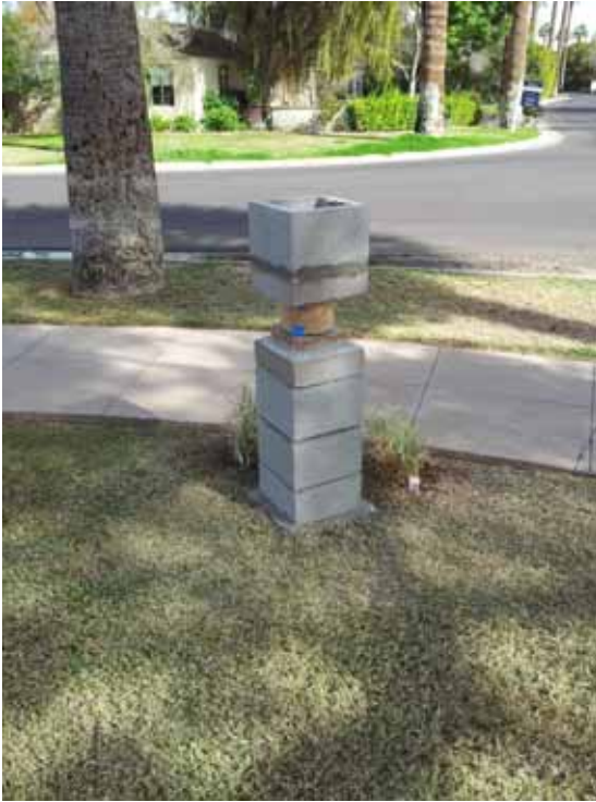
The column base is below the frost line.
